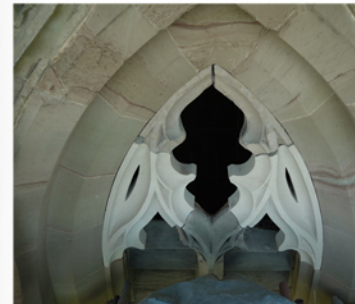
Repaired traceried opening
