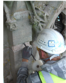
Cutting out stone for mortar repairs
