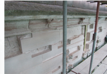
Cut-outs for masonry repairs
