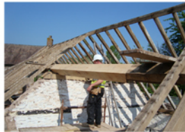
repairs to roof structure
