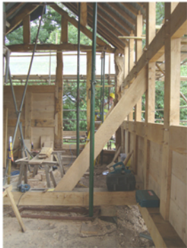
new timber frame wall
