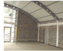
interior roof structure
