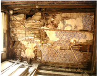
Typical view of internal wall frame and floors
